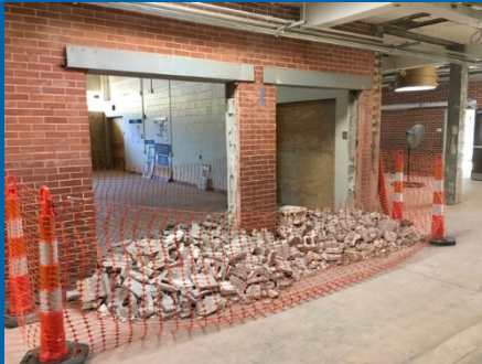
Demoed New Interior Openings and Installed Lintels
