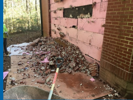
Demoing Exterior Brick at New Wall Opening
