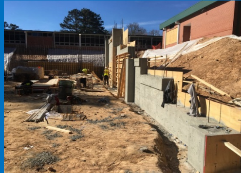
Stripping Forms at Concrete Retaining Walls at Gym
