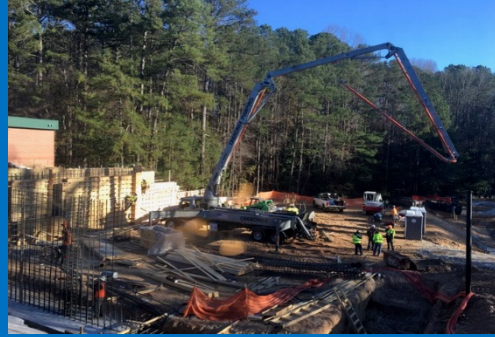
First Retaining Wall Pour at Gym Area
