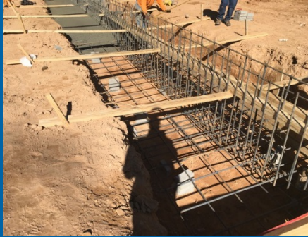
Pouring Footings at Gym Addition
