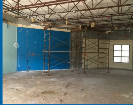
Installing Shoring to Demo Exterior Wall
